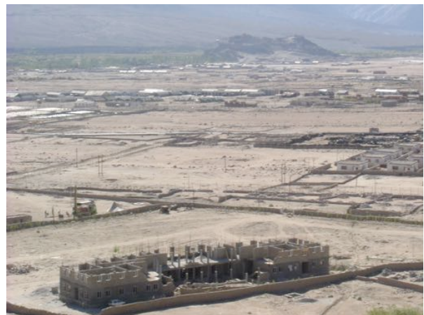
LHF Hospital under construction
