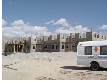
Second floor under construction
