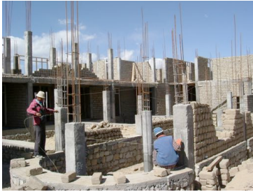
Ramp of the hospital
