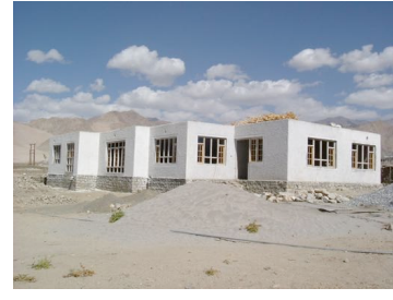
Guest house nearly complete
